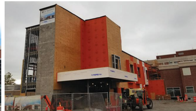
The new ICU, shown under construction in late September, will be larger and is expected to allow for more efficient, effective care.
